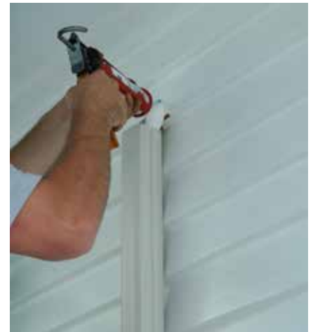
b. Applying sealant around pipework.
