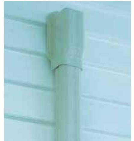
d. Cover in place over penetration and fully sealed to cladding.
