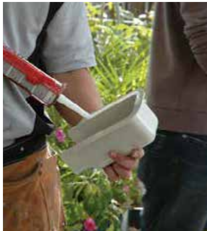
c. Applying sealant to cover.
