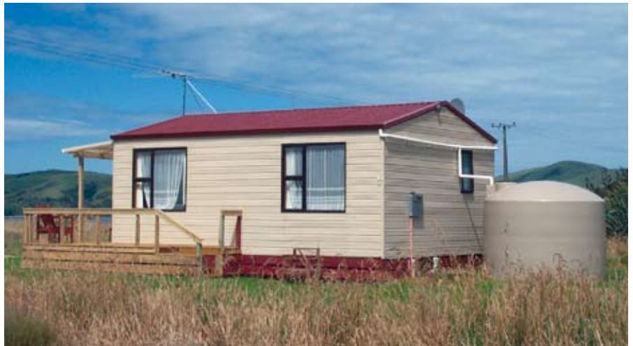
Collecting rainwater off roofs for drinking is popular in rural areas without town water supplies.
