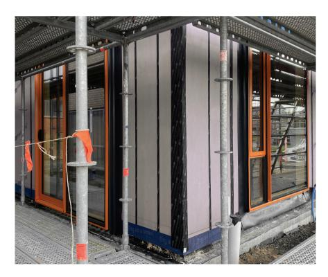
and is restricted from entering the building by the interior linings. Pressure moderation occurs within the assembly, negating the higher-pressure exterior driving force.
