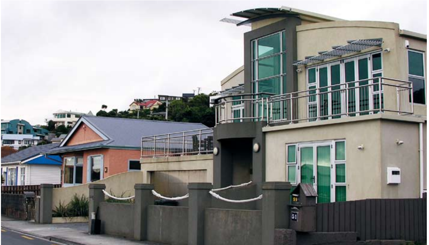
A modern house in the foreground which, like many new houses, has large windows and limited eaves. The older houses down the road have comparatively wider eaves and less windows.
