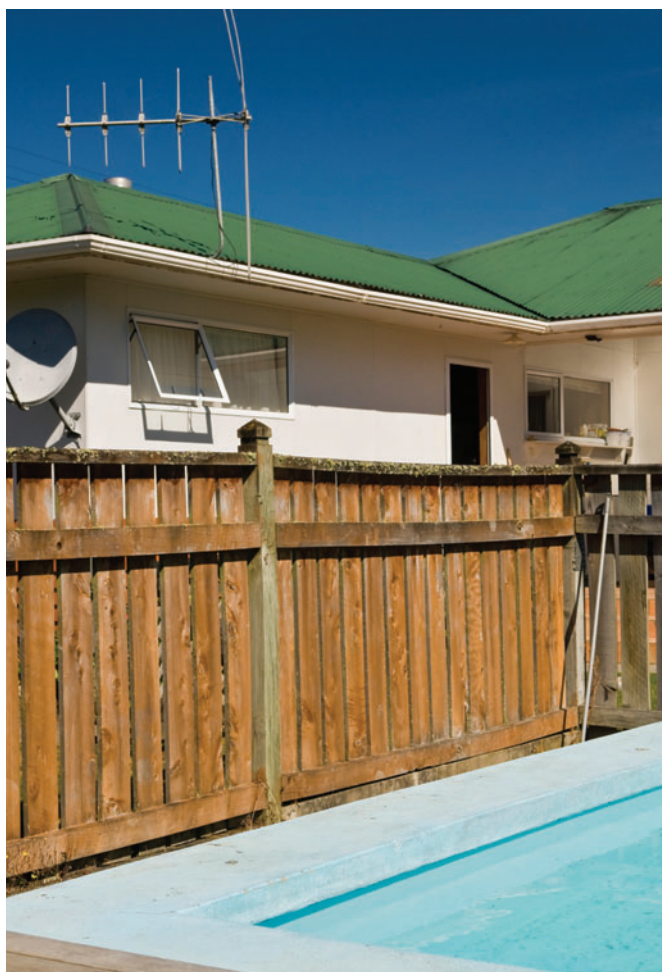
Fencing round a swimming pool must be permanent and comply with NZS 8500:2006.
