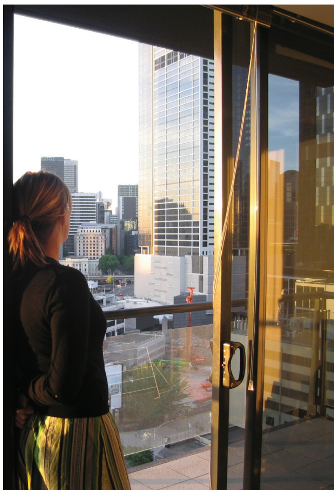
Grade A safety glass is required in places that may be subject to human impact, such as sliding doors and glass barriers.
